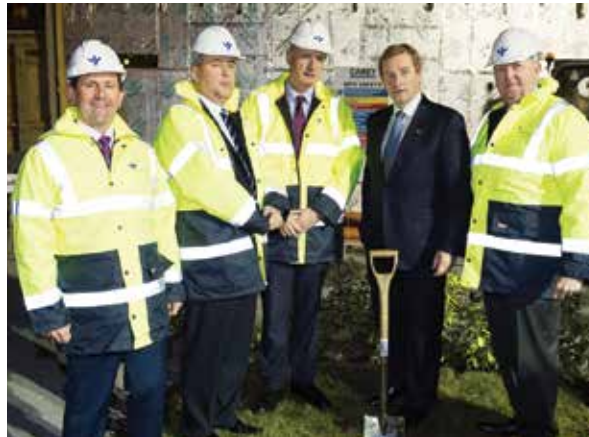
Pictured (l-r) at the turning of the sod on the new cardiology suite for Bon Secours Hospital in Galway were: Gerry Burke, CEO, Bon Secours Hospital, Galway; Bill Maher, CEO, Bon Secours Health System; Denis O'Sullivan, group head of projects, Bon Secours Health System; An Taoiseach, Enda Kenny; and Peter Lacy, chairman, Bon Secours Health System
